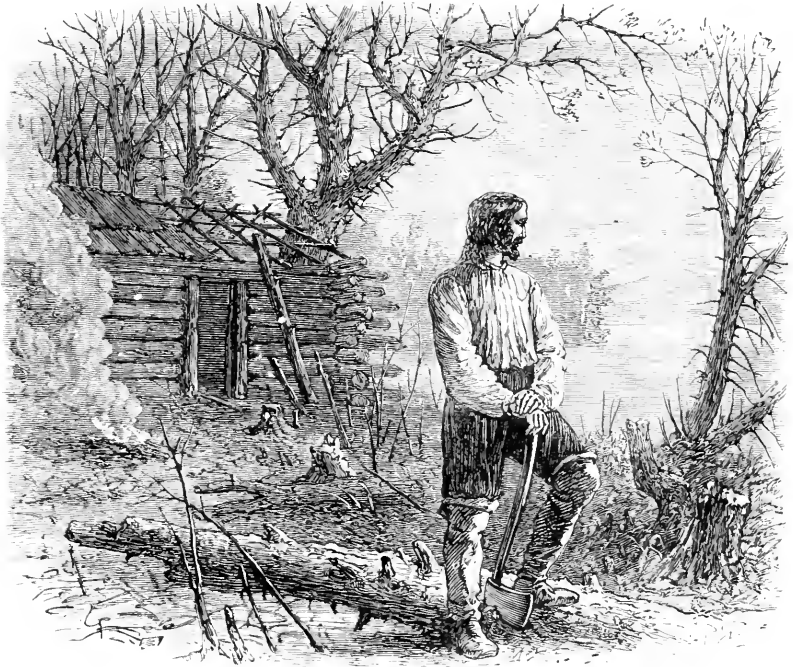
A SETTLER BUILDING HIMSELF A HOUSE AT PROVIDENCE.
